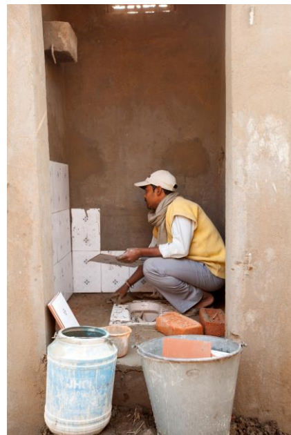
A new toilet is installed in Bihar. Photo credit: Kiran Thejaswi
